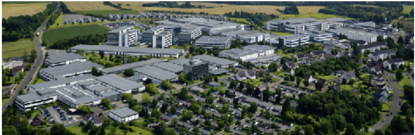
Headquarters Blomberg in Germany
